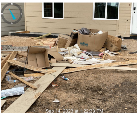
5. Riverdell- More construction trash littering the site. No trash dumpster on site. No SWPPP was located in the designated holder.
